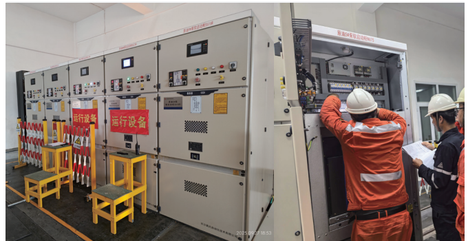
Large Oil Pumping Station Project
