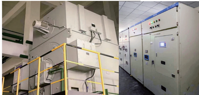
Baogang Group – Pellet Belt Roaster Desulfurization and Denitrification Upgrading Project
